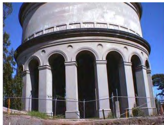
Water Reservoir, Bankstown
